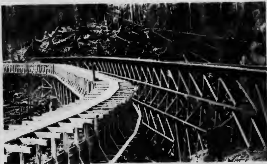
Vancouver Island Power Company Limited. Flume and Railroad on trestle.
